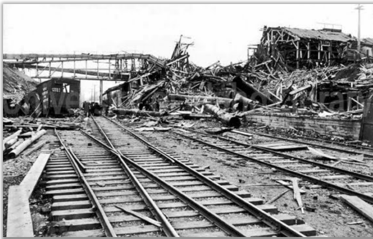
The mill at Wardner after the explosion. (Idaho State Historical Society)
